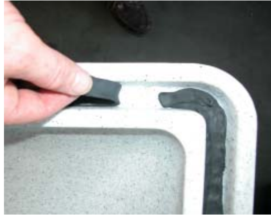
Step 2. Continue around vault with the same roll until you reach the corner you began with.
